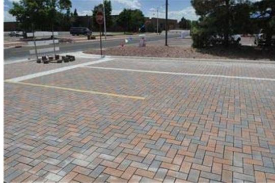
Construction crews are expected to complete a road project on Thule Street, next to McDonald's Restaurant, on Peterson Air Force Base by the end of August. Permeable pavers allow storm water to seep through the spaces between bricks into a subsurface detention area thereby reducing storm water runoff, which is part of Environmental Protection Agency and Department of Defense mandates for all federal development and redevelopment projects. (U.S. Air Force photo/Rob Bussard)
